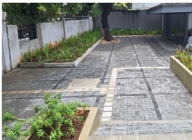
Figure 4 – POLI-UPE area, with permeable pavement in 2024.
