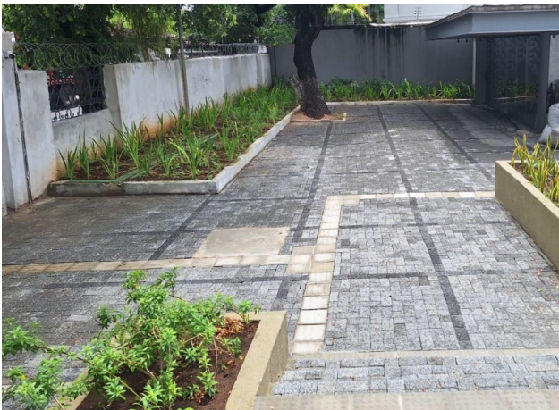
Figure 4 – POLI-UPE area, with permeable pavement in 2024.
