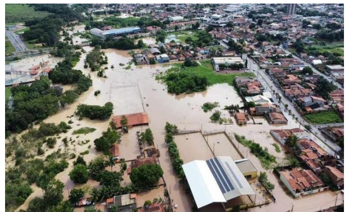
Figure 2 – Record of the overflowing of the Uraim River in Paragominas, PA, March 2024.
