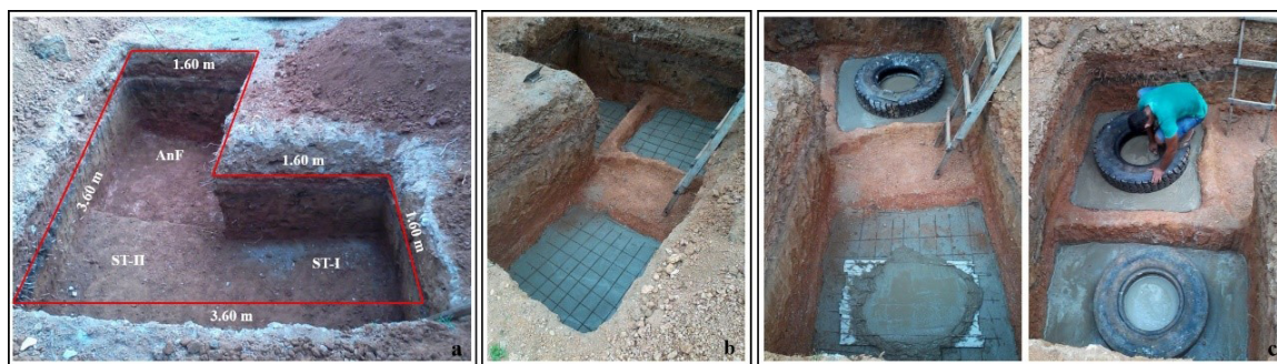
Figure 6 – Excavation of the trench for accommodating the TIRE-ATS (A); concrete piece at the bottom of the trenches (B); fixation of tires at the base of the units (C).
