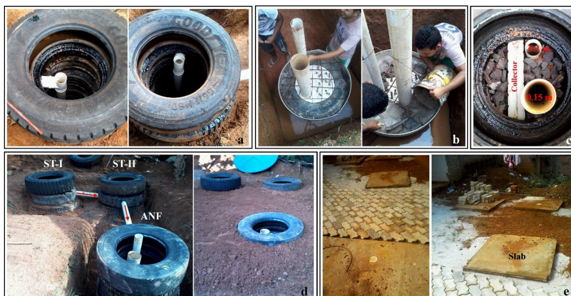
Figure 7 – Assembly and fixation of ST-I and ST-II (A); arrangement of pipes, construction of the concrete plate (false bottom) (B); filling of the AnF with gravel and installation of the treated sewage adhesive tube (C); drilling of the units and final arrangement (D); closure and system design (E).
